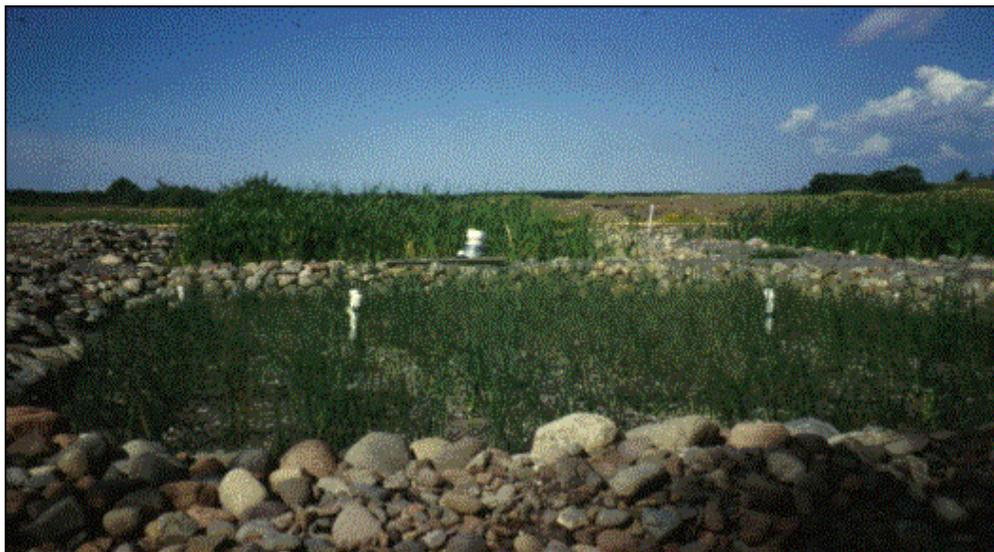
**Figure 3. One of the NERCC 2-cell constructed wetland treatment system after the first growing season in 1996.**
