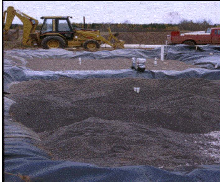
**Figure 2. The placement of pea rock over limestone in the second-cell of the constructed wetlands at NERCC in the fall of 1995.**
