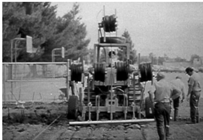
Figure 7. Installation of drip tubing
