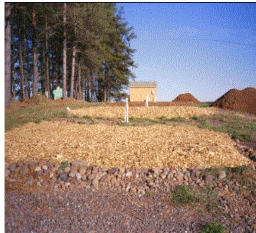
**Figure 3. Installation of the pressure distribution network and the completed sand filters covered with wood chips at NERCC.**
