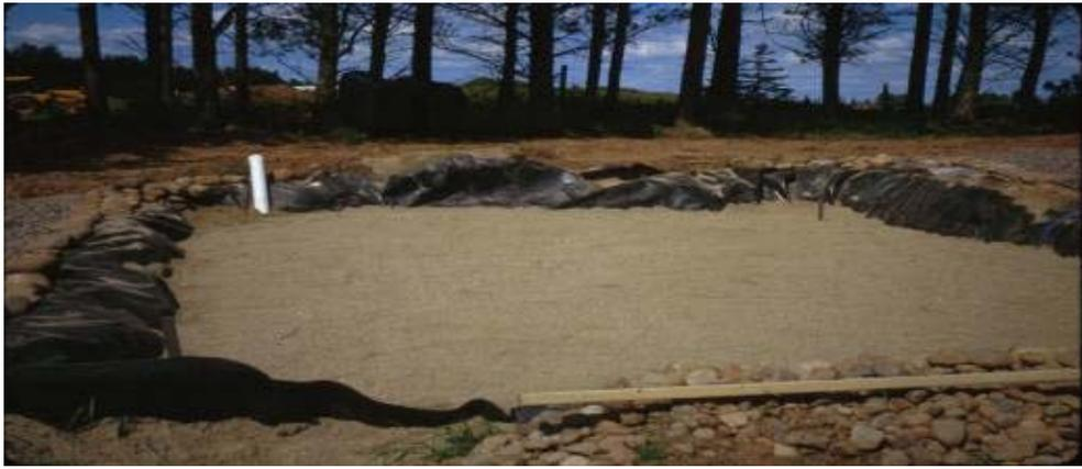
**Figure 2. A single-pass sand filter being constructed at NERCC showing the top of the media before completion of the distribution network and final cover.**
