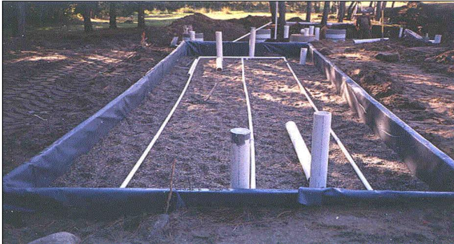
**Figure 4. Construction of a recirculating sand filter at the Iron Range Resources and Rehabilitation Board (IRRRB) office building in Eveleth showing the pressure distribution network and observation pipes.**
