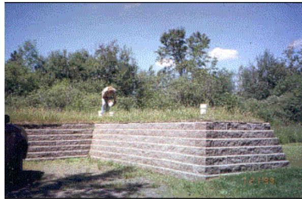
**Figure 1. Single-pass sand filters for two different homes on small lake lots: one system above the ground surface(using locking blocks) due to high ground water; the second system is below the surface in the grassy area (with well-drained soils) next to the garage.**
