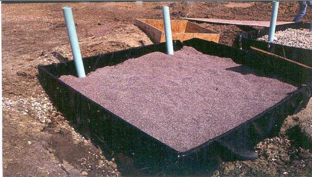
**Figure 5. The Lake Washington recirculating sand filter, designed for a single-family home, shows the support framing, liner material and top of the sand media. The PVC pipes are clean-outs.**
