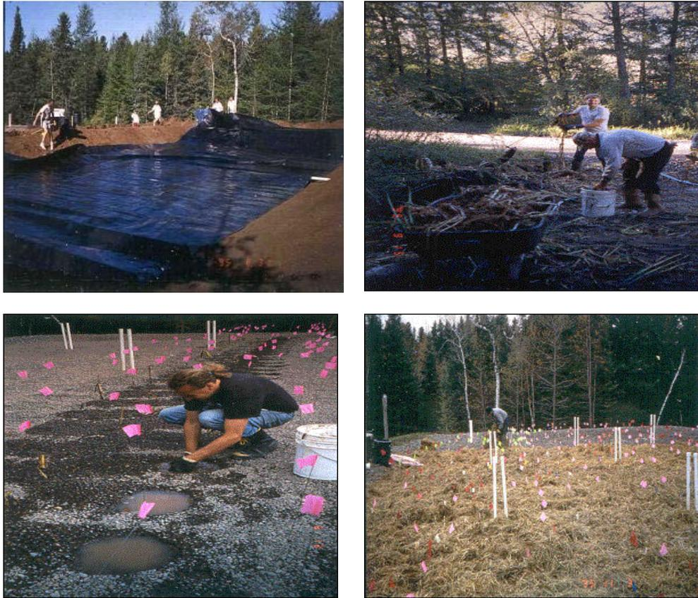
**Figure 2. Construction activities included: placement of a liner, preparation of cattails for planting, placement of pea rock and planting cattails, and insulating it with mulch.**
