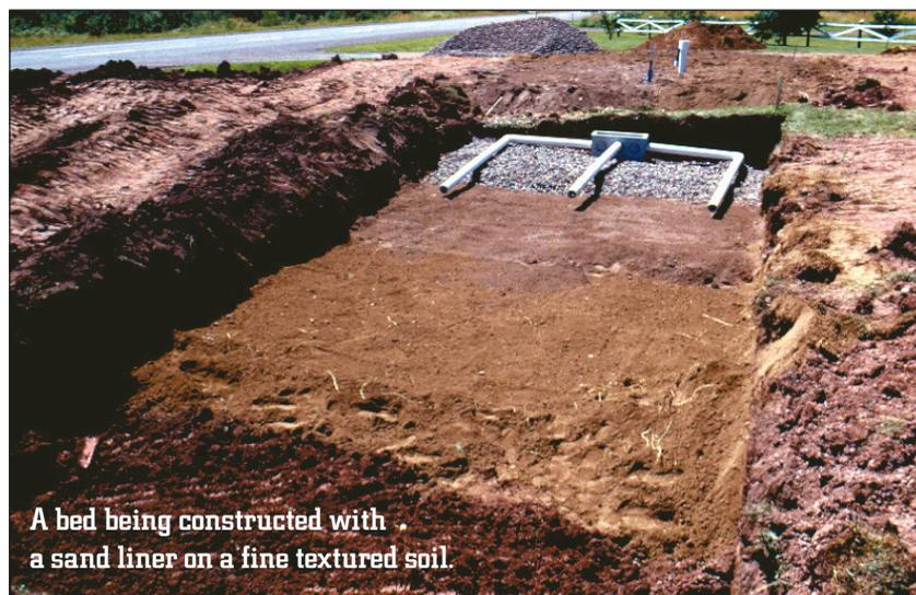
**A bed being constructed with a sand liner on a fine textured soil.**
