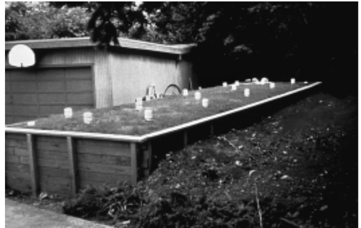
Figure 1. Single-pass sand filter
