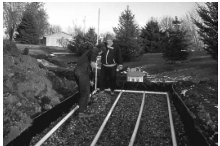
Figure 2. Low-rate sand filter being installed
