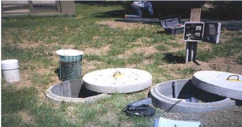
**Figure 7. Routine maintenance of peat filter systems is needed to ensure that they are working properly and to prevent pre-mature failure of the system.**
