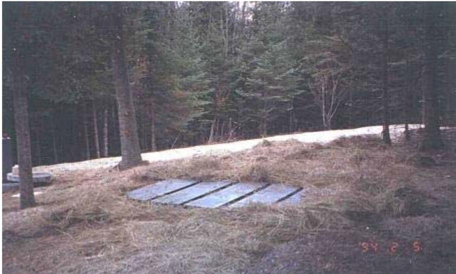
**Figure 8. A peat filter module coupled with an “at-grade” soil dispersal system is used to treat septic tank effluent and disperse it into the natural soil on this lakeshore lot.**
