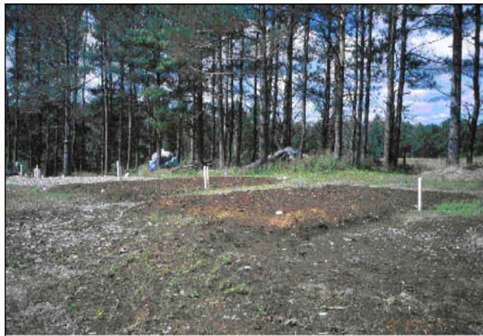
**Figure 4. A view of two identical in-ground peat filters each sized for a single family home at NERCC.**
