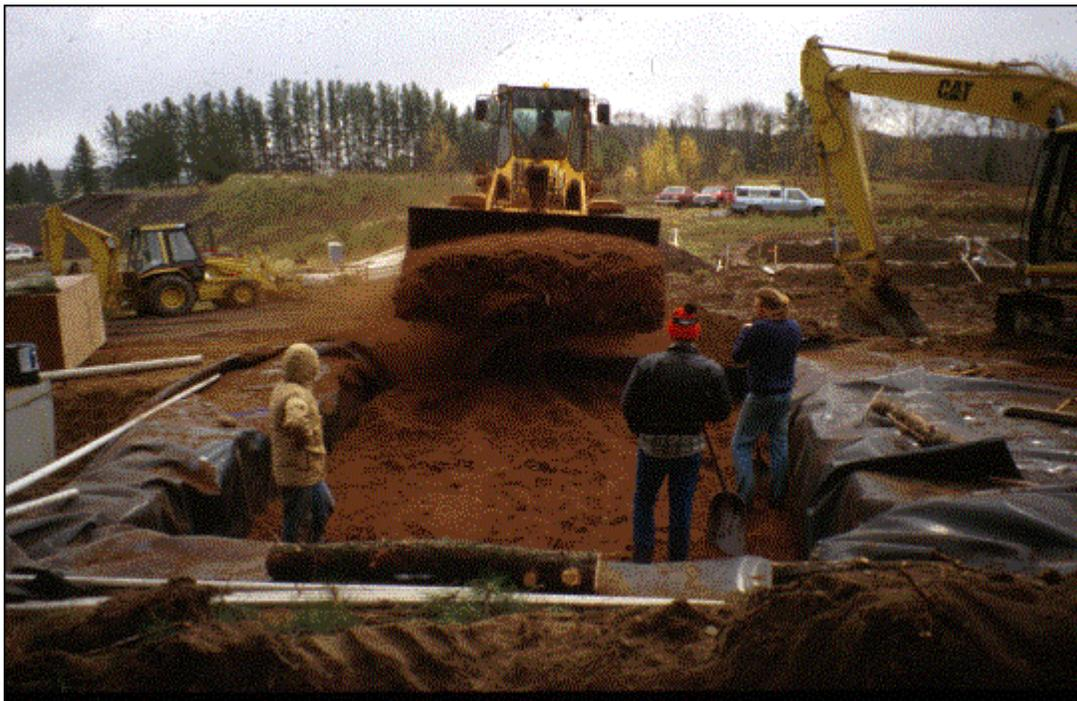
**Figure 2. Construction of an in-ground single-pass peat filter at NERCC.**
