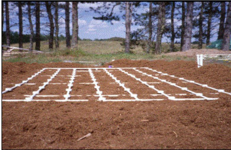
**Figure 3. Placement of the pressure distribution network in a peat filter at NERCC.**
