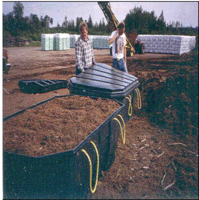
**Figure 5. An aboveground view of modular peat filters showing the distribution network, peat over the network, and the cover being placed over the module.**
